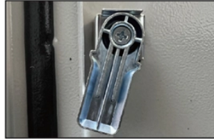
Strengthen door locks
